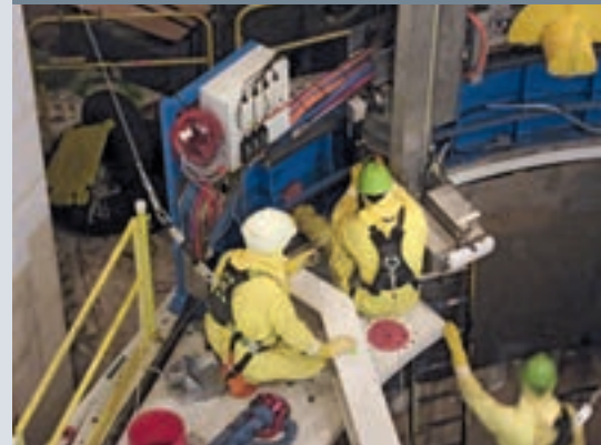
Installation of the flame cutting system
