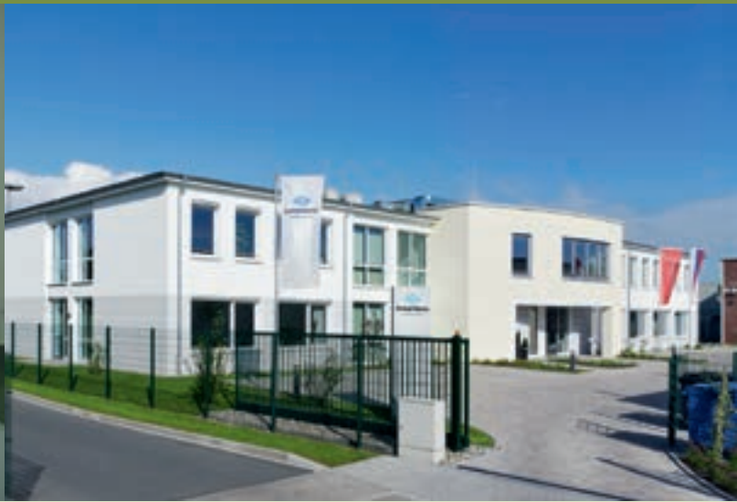
STS building in Lünen, Germany
