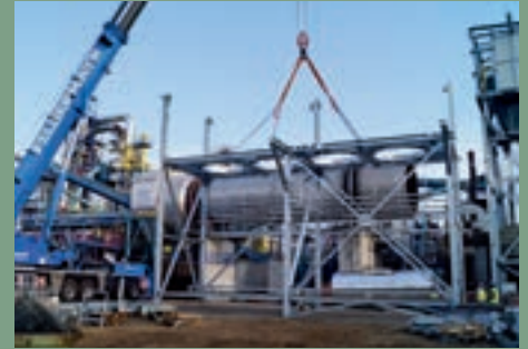
Final inspection before the new structure for the cyclones is installed.
