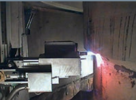
View of the first L-cut from the outside
