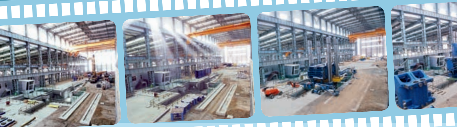
Installation process of 500 MN press in a time-lapse film (from left to right)
