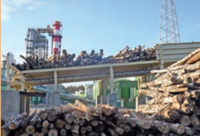
Material feed – from debarker to chipper
