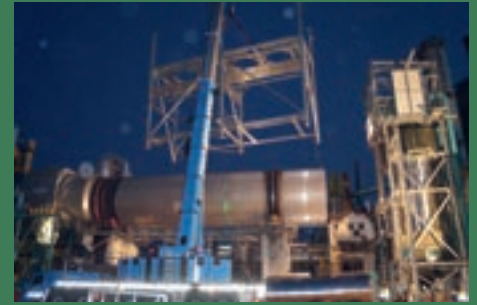
...to the new foundations directly behind the Büttner drum dryer
