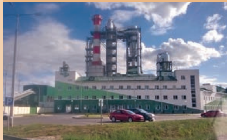
Gomeldrev location – an ambitious project
