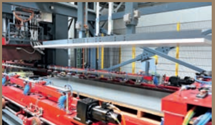
Placing the panel after edge finishing
