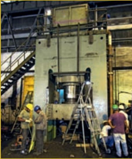
20 MN press prior to the modernization
