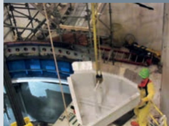
Complete installation of the slag pans
