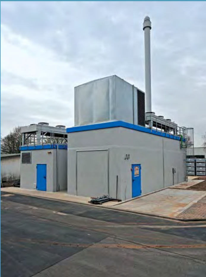
The complete cogeneration unit – plenty of power in a small space
