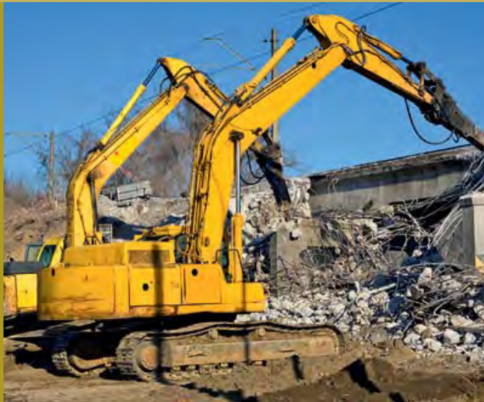
Demolition of former military buildings, e. g., residential buildings, fuel depots
