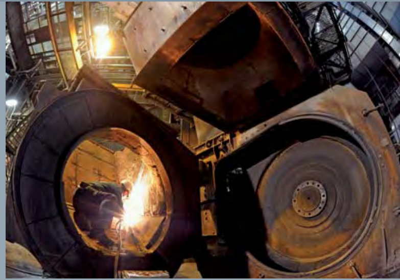
Cutting works at the exhaust system (photo: Andreas Seidel, Chemnitz)
