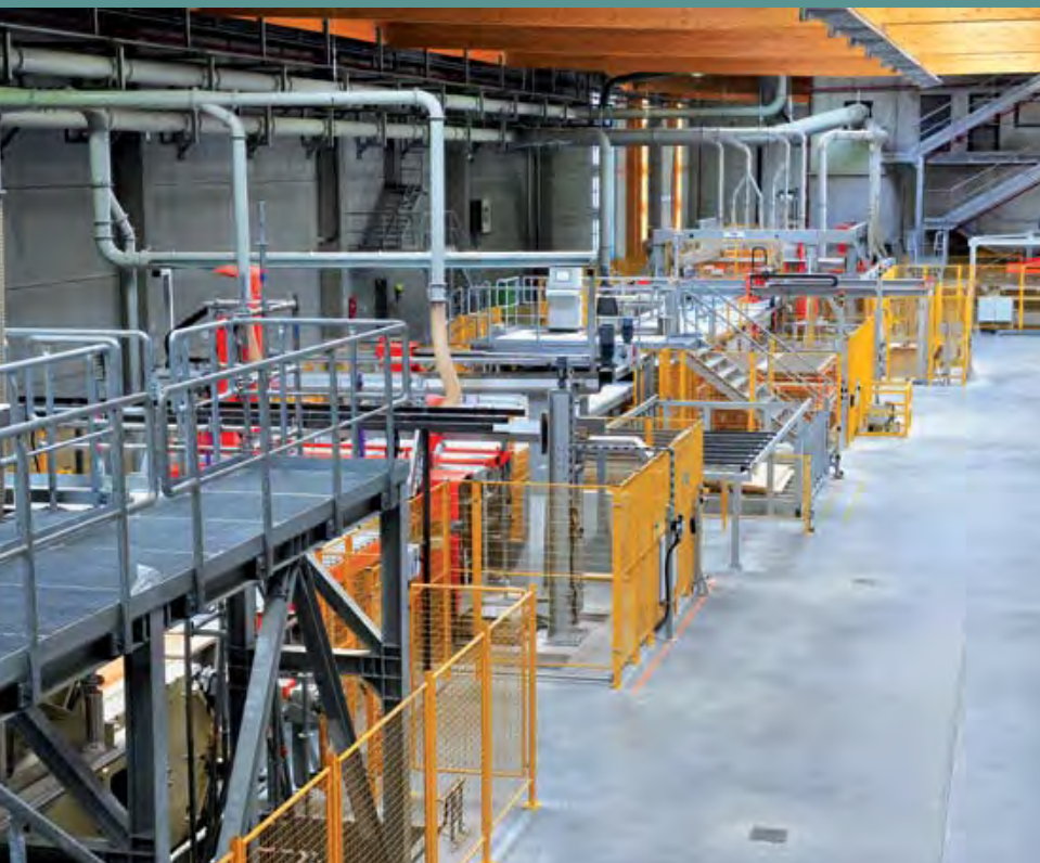
Saw system after mat-forming
