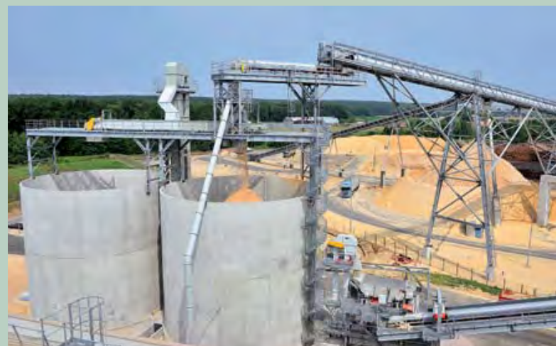
Chip silos with discharge system and oscillating screen
