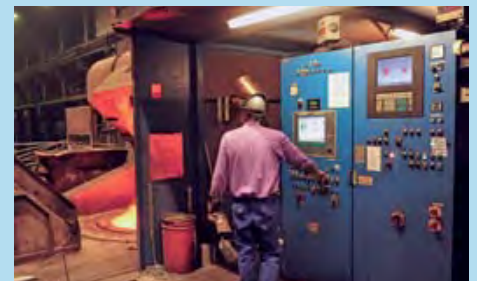
Modern induction furnaces for the melting and holding of the molten iron are used in the melting shop
