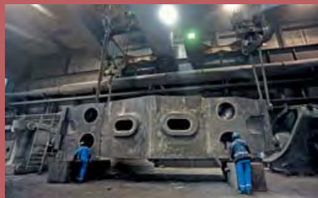
Left: Lift out of the lower press beam
