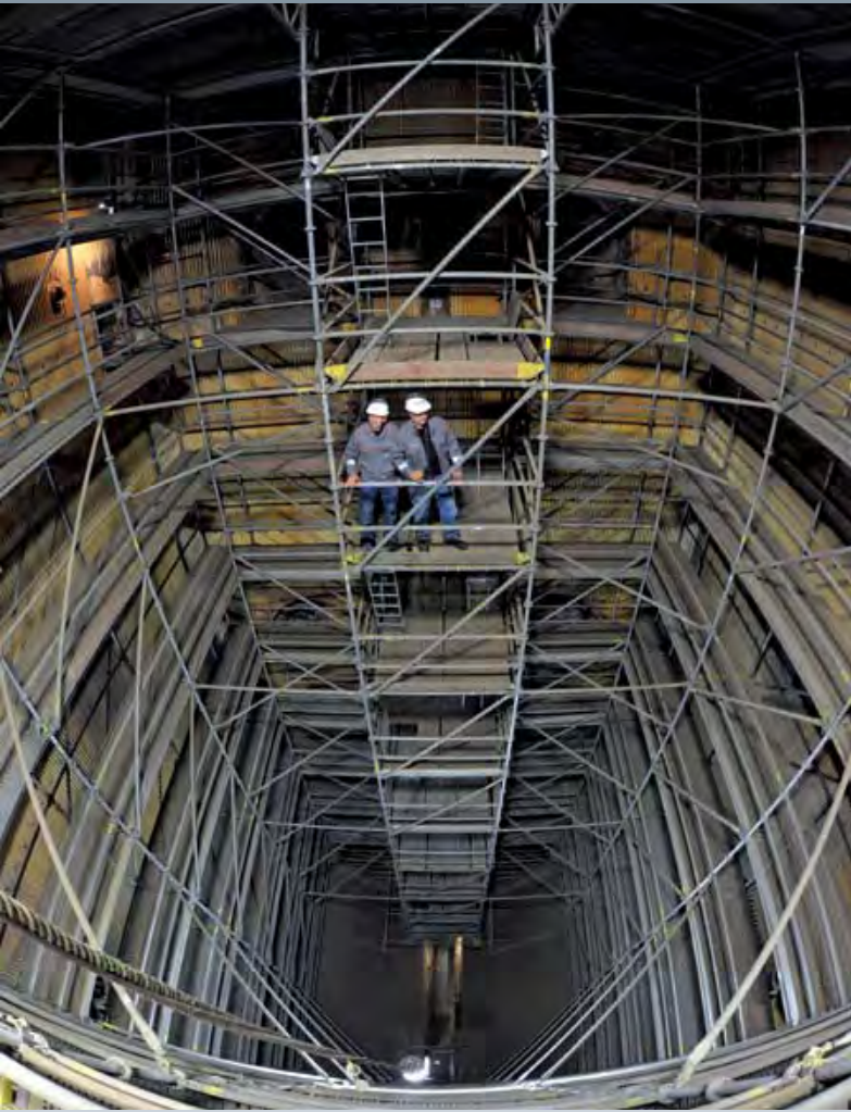
Scaffolded for inspection: the boiler house (photo: Andreas Seidel, Chemnitz)
