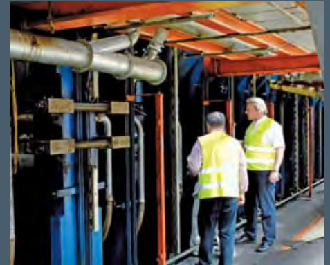
Inspection of the retrofitting works by Siempelkamp employees
