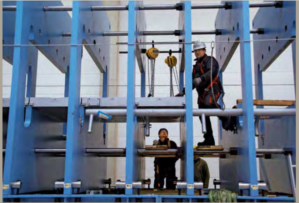
Installation of pressure distribution plates
