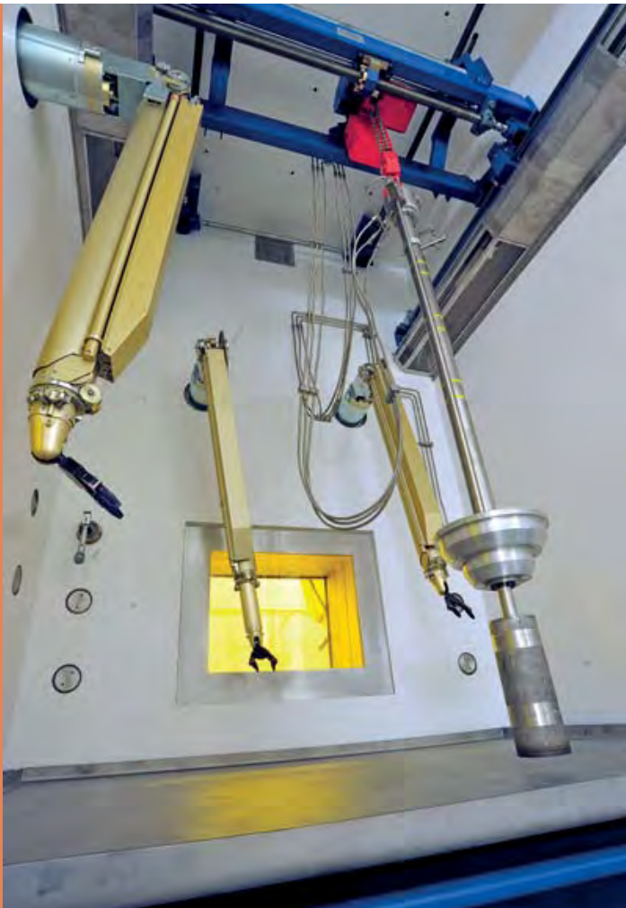
The cell crane has gripped the tamping tool
