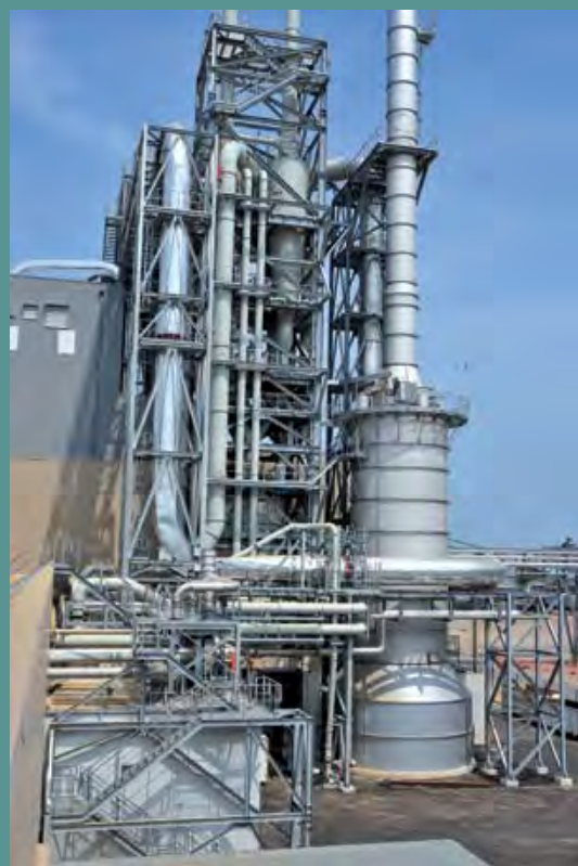
Dryer with wet electrostatic precipitators
