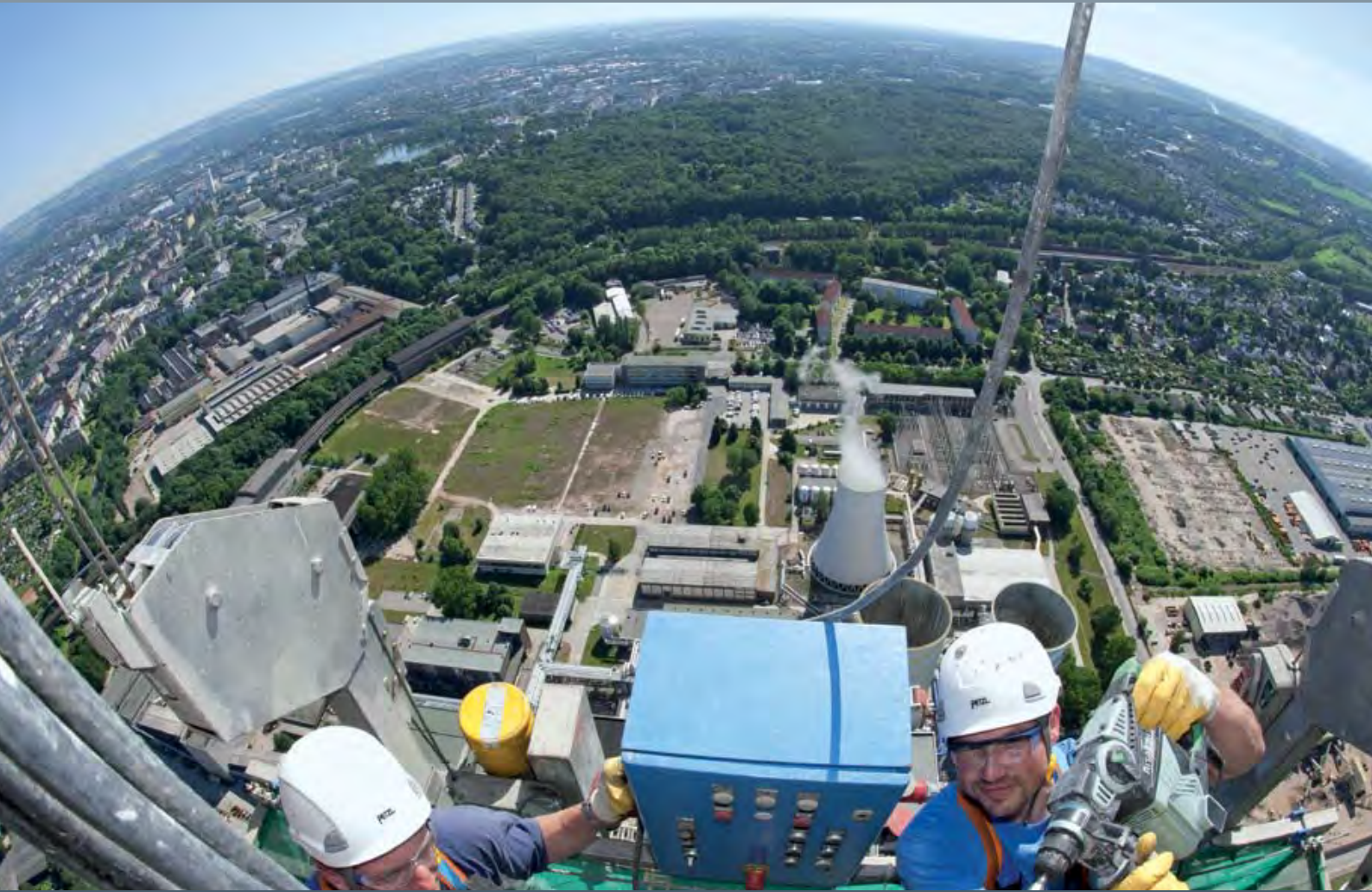
Provision of power and heat for Chemnitz viewed from the chimney of the power plant (photo: eins energie in Saxony)
