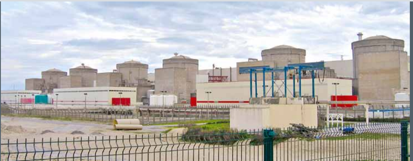
The French nuclear power plant Gravelines with six units of 910 MW each
