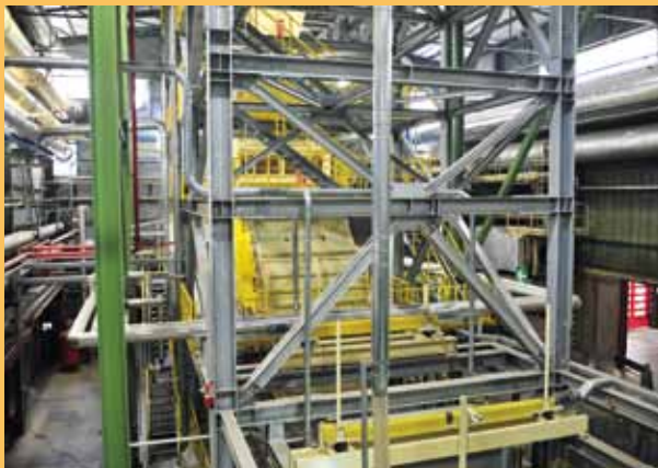
Steel structure for the forming line
