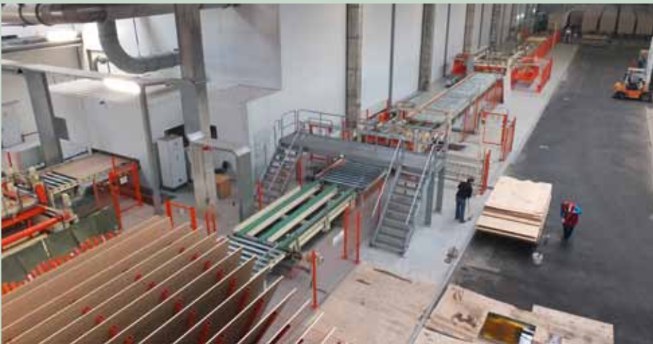
Left: Connection to the storage
