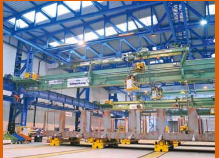
Section equipment in production hall 11 of the MEYER WERFT laser center
