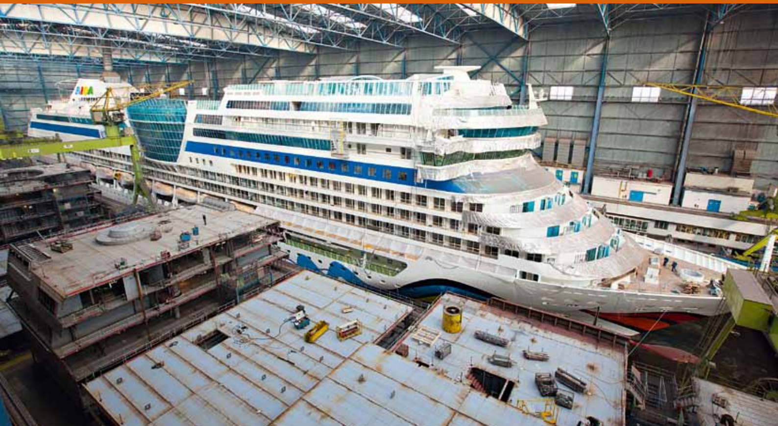
The cruise ship AIDamar on the building site deck (photo: MEYER WERFT)
